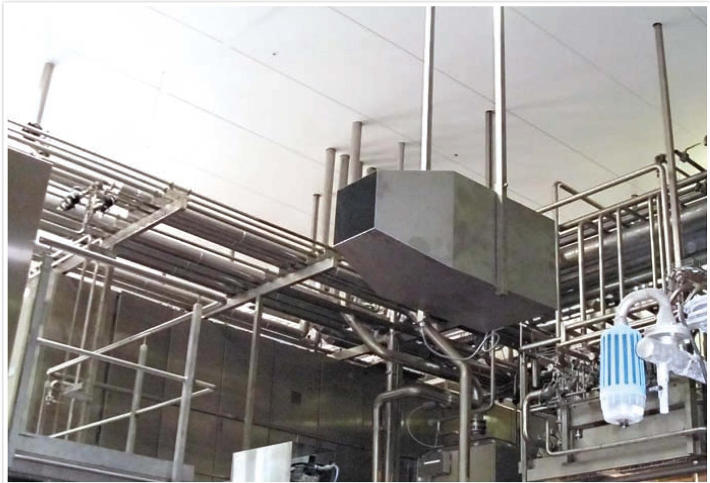
**Air circulation unit using the Just Air concept**
