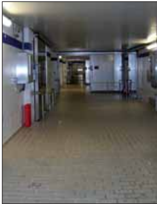
This entire hall area is flooded by degerminated air
